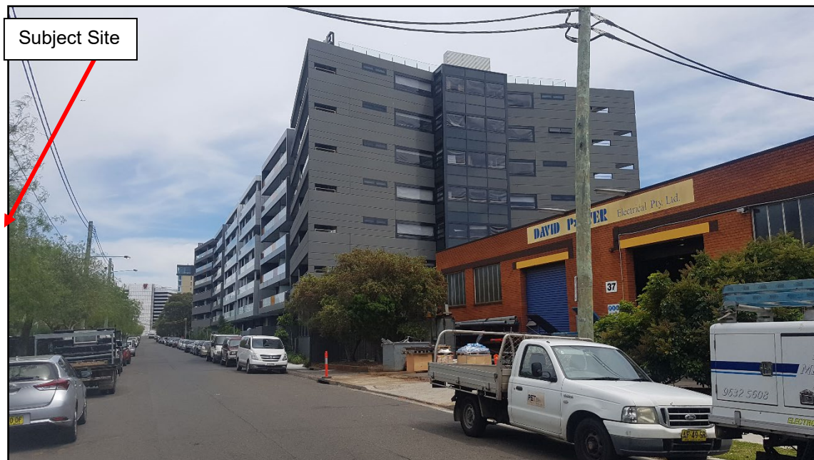
Figure 9: Development to the north of the subject site, on the northern side of Baxter Road, looking west along Baxter Road
